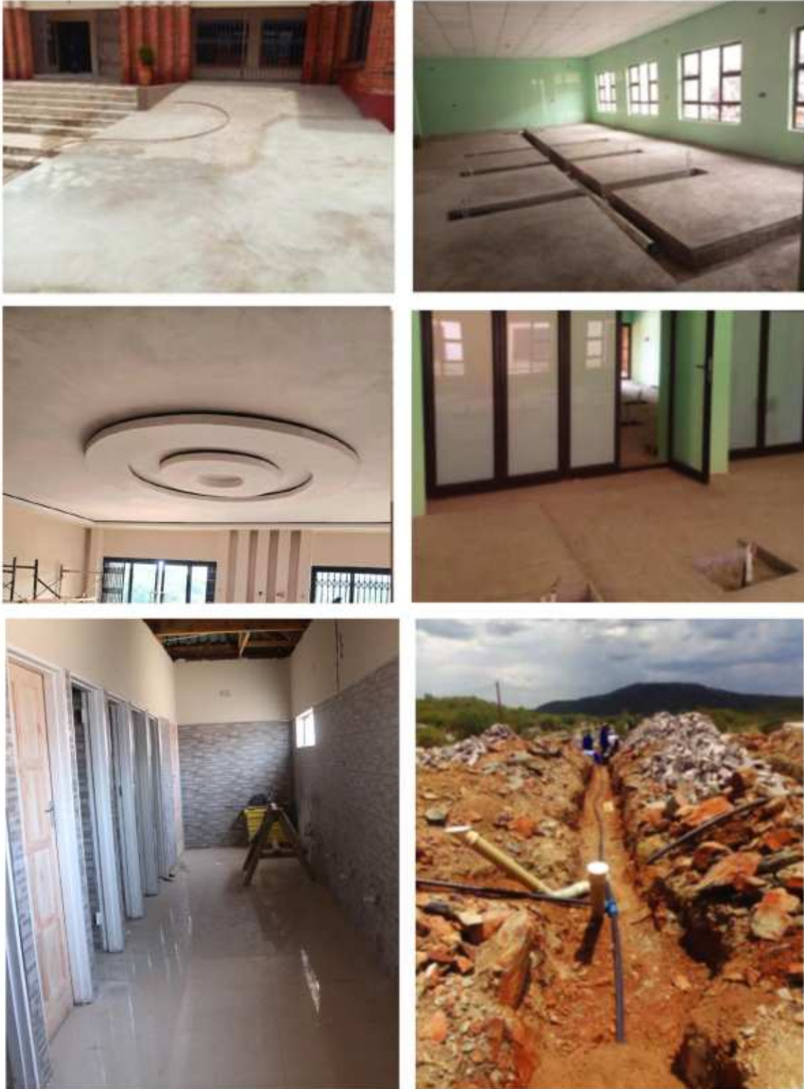
Agro-Innovation construction progress, featuring exterior, interior and ceiling installations
