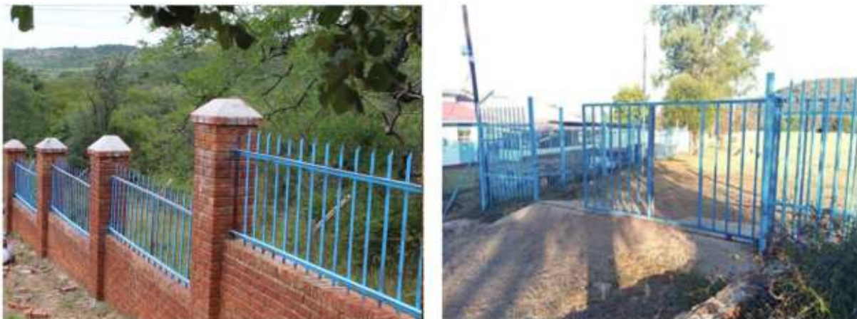
Construction progress of the Palisade
