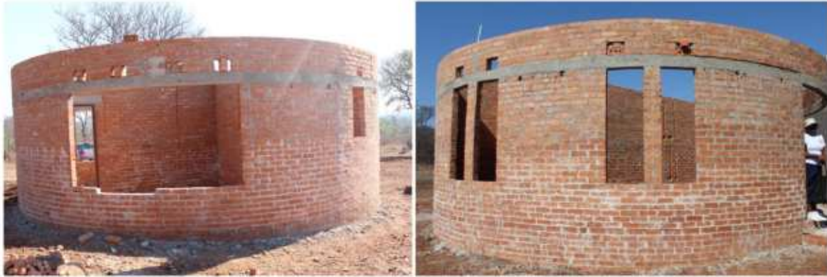
Construction progress of the Chalets
