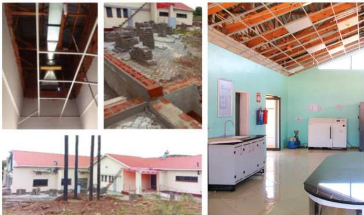
Construction progress of the Engineering Laboratory and Innovation Complex, showcasing exterior, interior and structural developments.
