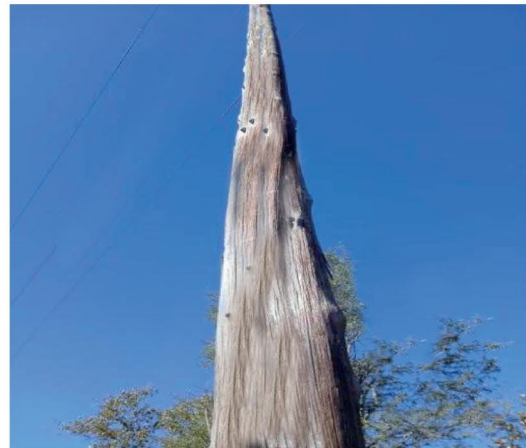
New powerline pole
