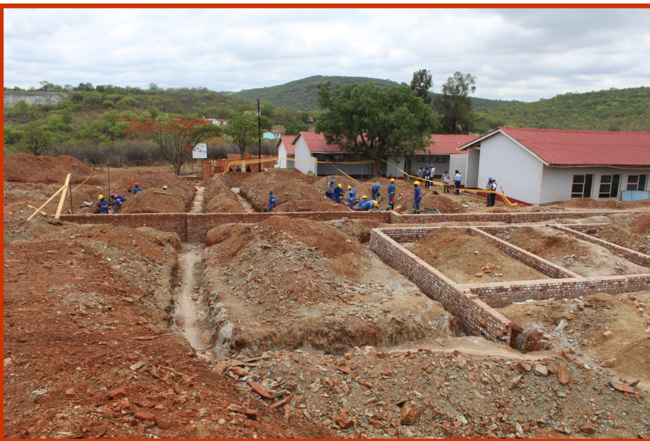
Part of the foundation construction of the Mining and Engineering Laboratory at Epoch Mine Campus
